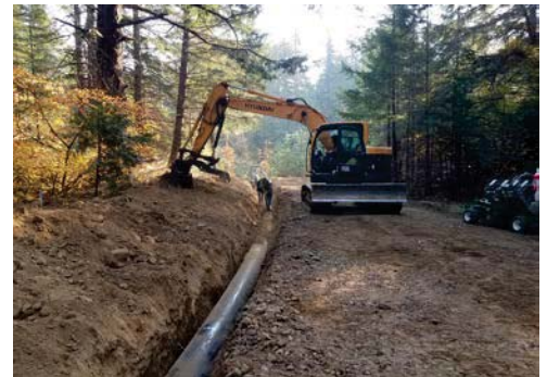
Installing 18-inch HDPE pipe. Photo by Carly Lemon
