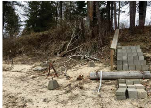
Example of mass bank failure on the Pend Oreille River.
