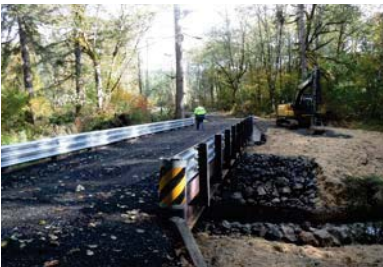
Newly installed bridge over King Creek. Photo by Kelly Verd
