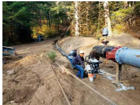
Installing the filter. Photo by Carly Lemon
