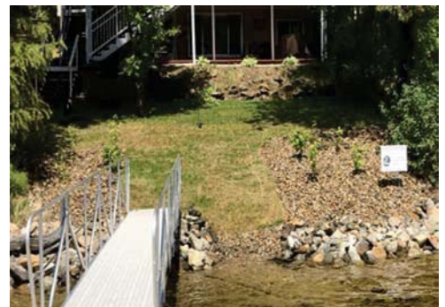
Bank stabilization practices on Davis Lake. An example of maintaining aesthetics while addressing erosion.
