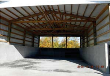
Dry stack for safe waste storage on a horse farm. Photo by Kelly Verd
