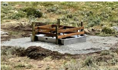
Livestock watering trough reduces impacts on nearby surface waters and improves grazing in the Okanogan Highlands. Photo by Mindy Untalan
