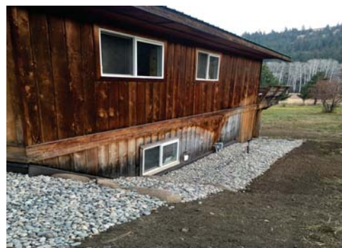
Landowner participated in a home-hardening cost share program to add three to five feet of gravel perimeter around the home. Photo by Mindy Untalan
