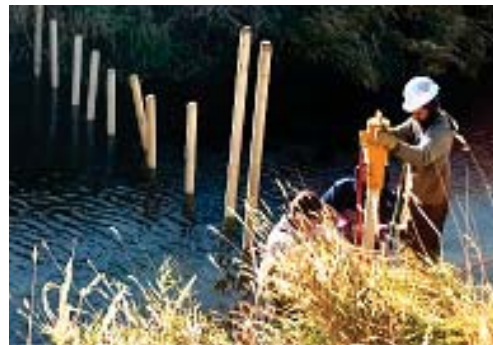
U.S. Fish and Wildlife installing Beaver Dam Analogs. Photo by Jeff Kuhlmann, USDA Natural Resources Conservation Service
