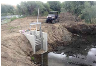
Benton County Voluntary Stewardship Program funding was used to install water control structures at Mast Farms to increase floodplain functionality. Photo by Bob Montgomery, Anchor QEA
