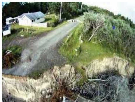
North Cove – before.
