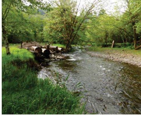
Instream wood structure creates fisheries habitat, improves water quality, and protects streambank so trees can establish.
