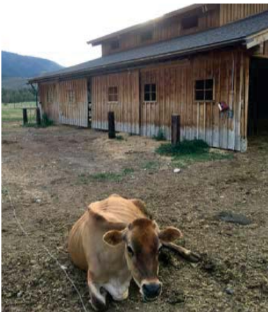
Newly installed gutters on a micro-dairy as part of a dairy nutrient management plan project in the Methow Valley. Photo by Allisa Carlson
