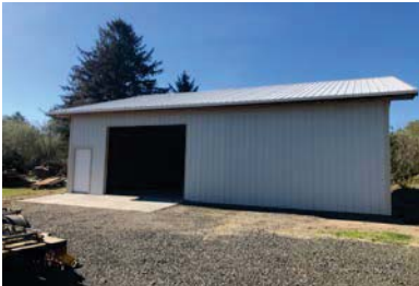
Chemical storage and mixing sheds – a new practice opened up through the Voluntary Stewardship Program (VSP) for cranberry farmers' water quality program. Photo by Courtney Hagain
